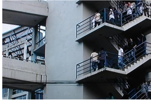
Figure 9. The evacuates walked through the emergency stairs outside the building (on the right) and the connecting bridge to the next to building (on the left).
