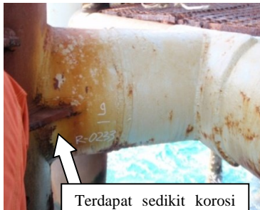
Gambar 15 Tampak dekat clamp support [8]
