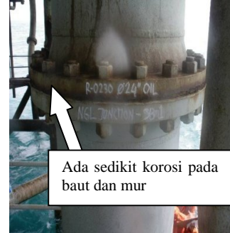
Gambar 17 Tampak dekat flange Line B [8]
