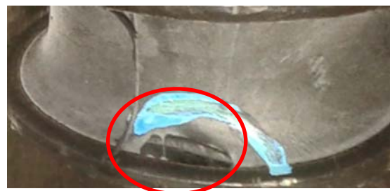
Gambar 3. close figure crack bushing rear suspension
