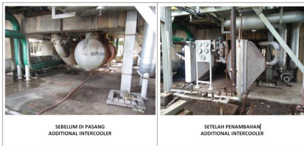
Gambar 9. Penambahan Additional Intercooler
