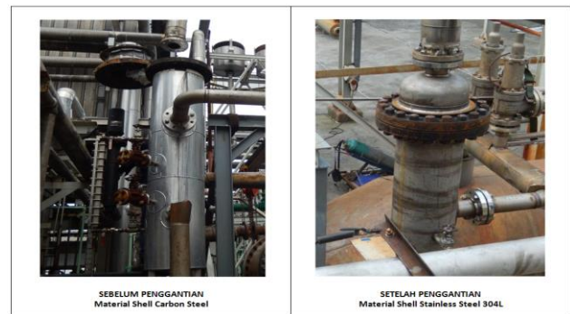
Gambar 6. Penggantian Equipment Equipment Mist Eliminator (2-V-001)
