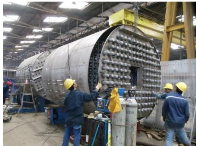
Gambar 3. Equipment Dalam Proses Refurbishment
