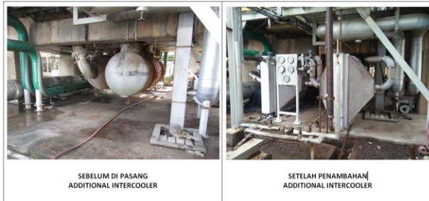
Gambar 9. Penambahan Additional Intercooler
