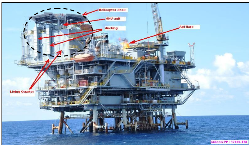
Gambar 1: HVAC- Kakap Field Platform –Star Energy – Natuna
