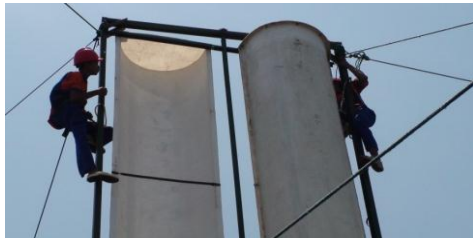
Gambar 3. Proses assembly kincir angin
