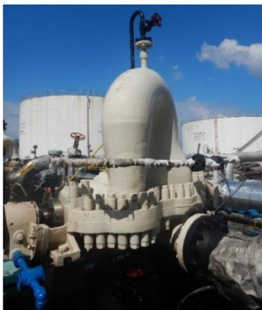
Gambar 1. Centrifugal feed pump
